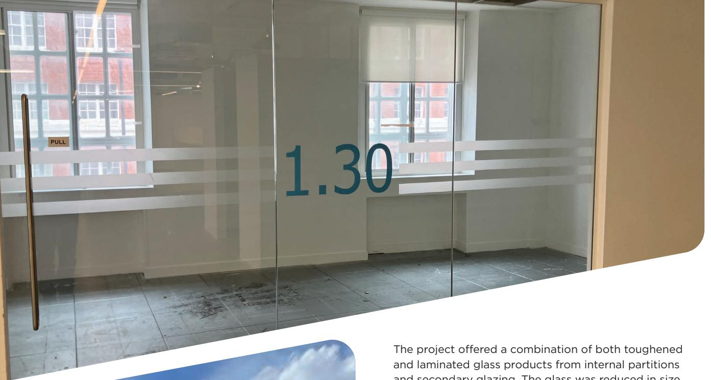
The project offered a combination of both toughened and laminated glass products from internal partitions and secondary glazing. The glass was reduced in size on site maintaining the necessary clean quality controls, placed into Saint-Gobain Glass cullet bags, collected by Glassolutions Thurrock and then returned to Saint-Gobain Glass on a return trip vehicle.
